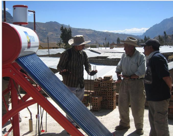
A solar water heater being installed at a hostel in Chivay, Peru.
